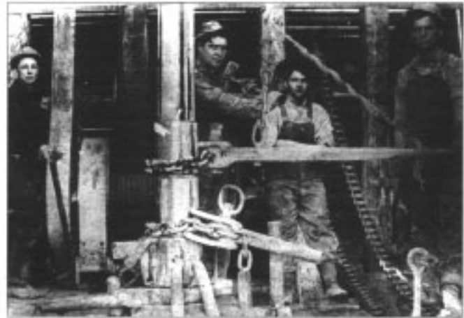
Early wells were drilled with nothing installed above the drill pipe to control pressure.
